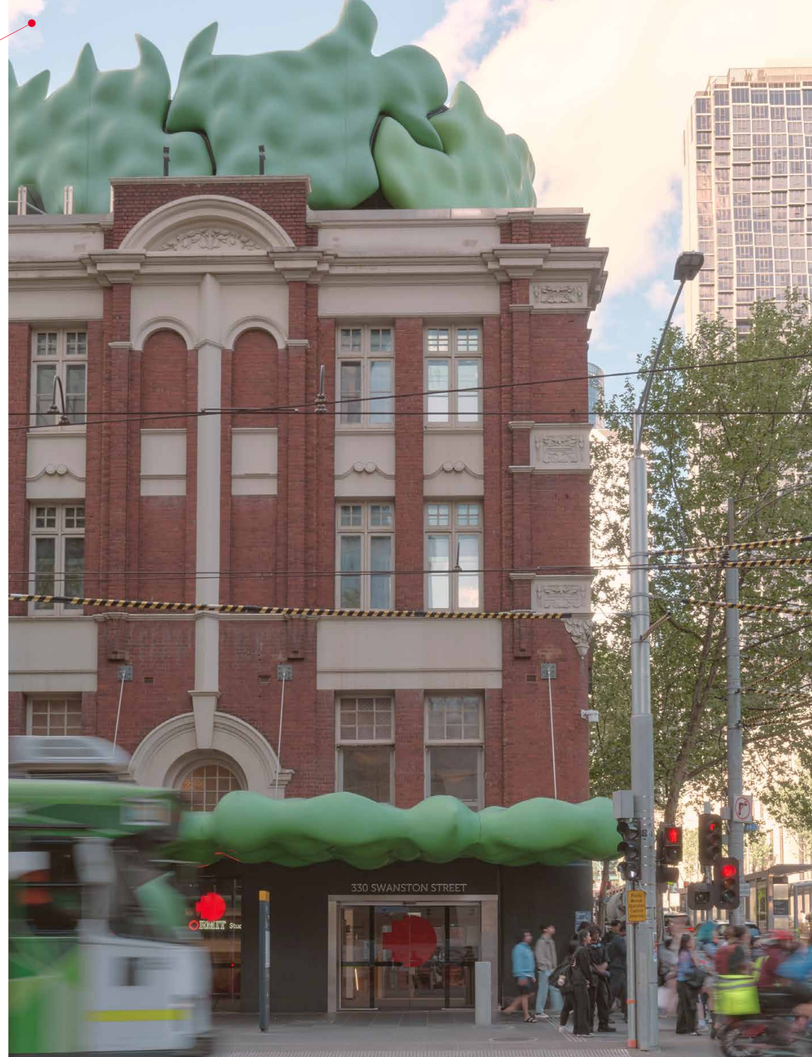
Building 22, RMIT City
